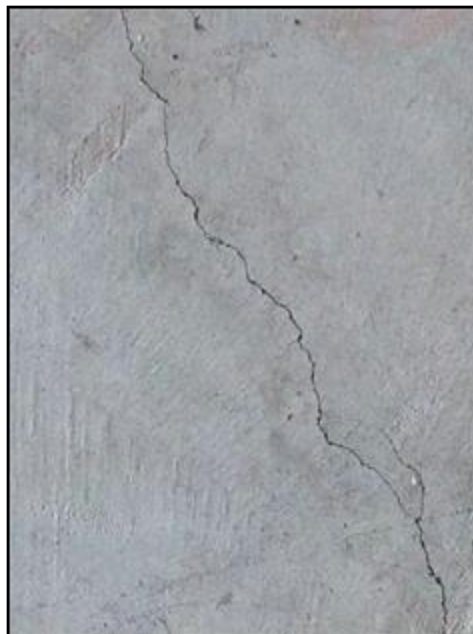
15. Typical minor cracks
