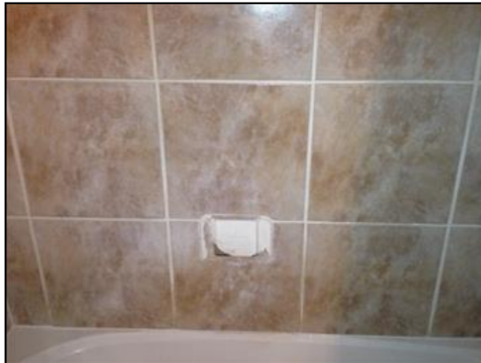
25. Tile loose, broken or missing tile
