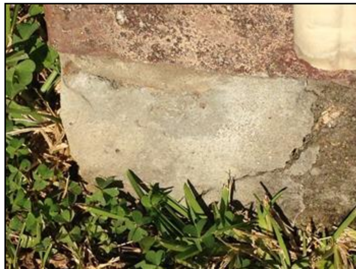
16. Spalling, crumbling or broken material
